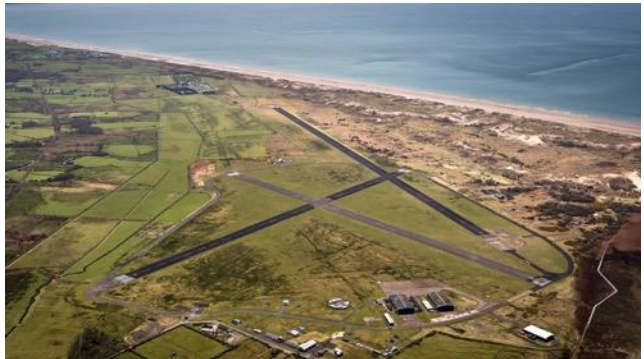
Fig. 1d - aerial view looking south
