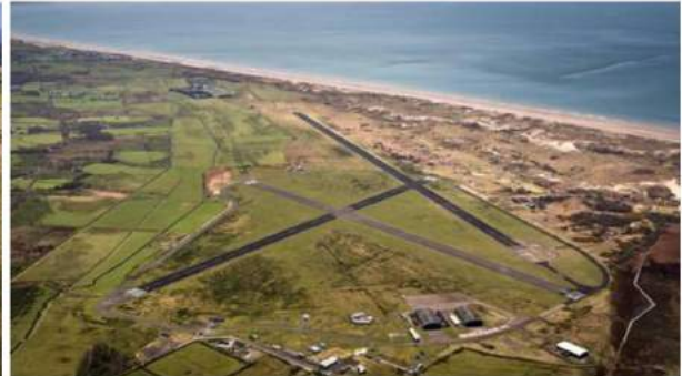
Fig. 1d - aerial view looking south
