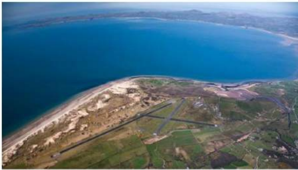
Fig. 1a - aerial view looking west
