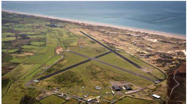
Fig. 2d - aerial view looking south
