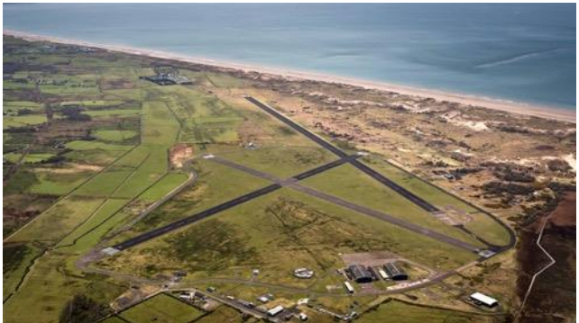
Fig. 1d - aerial view looking south
