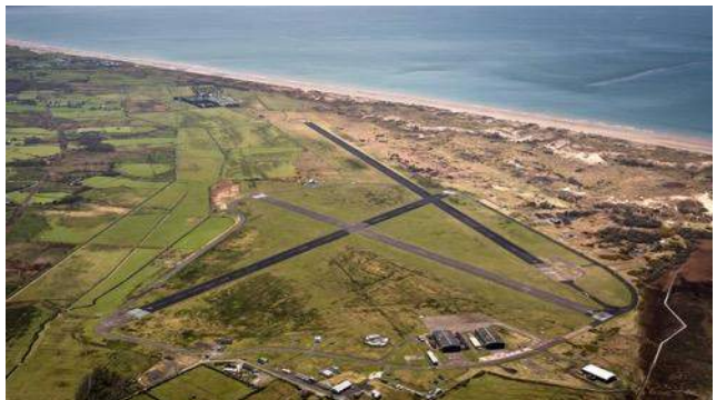
Fig. 1d - aerial view looking south
