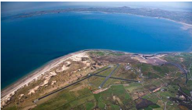
Fig. 1a - aerial view looking west
