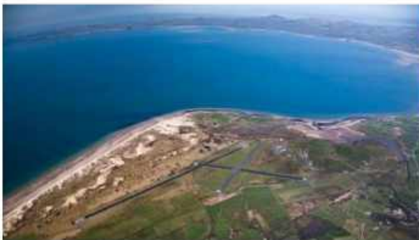
Fig. 2a - aerial view looking west
