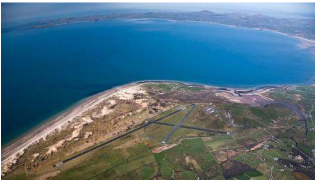
Fig. 1a - aerial view looking west
