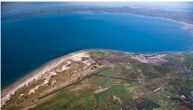
Figure 1a - aerial view looking west
