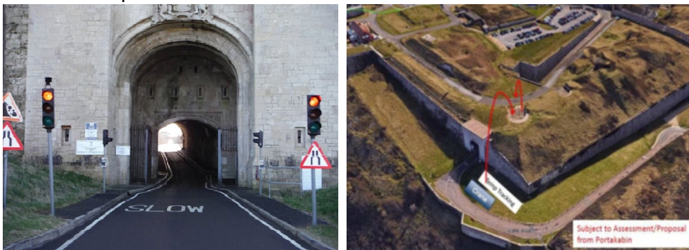
Figure 11 The narrow entrance tunnel into HMP Verne and the lorry offload plan via craneage necessary to avoid it.
