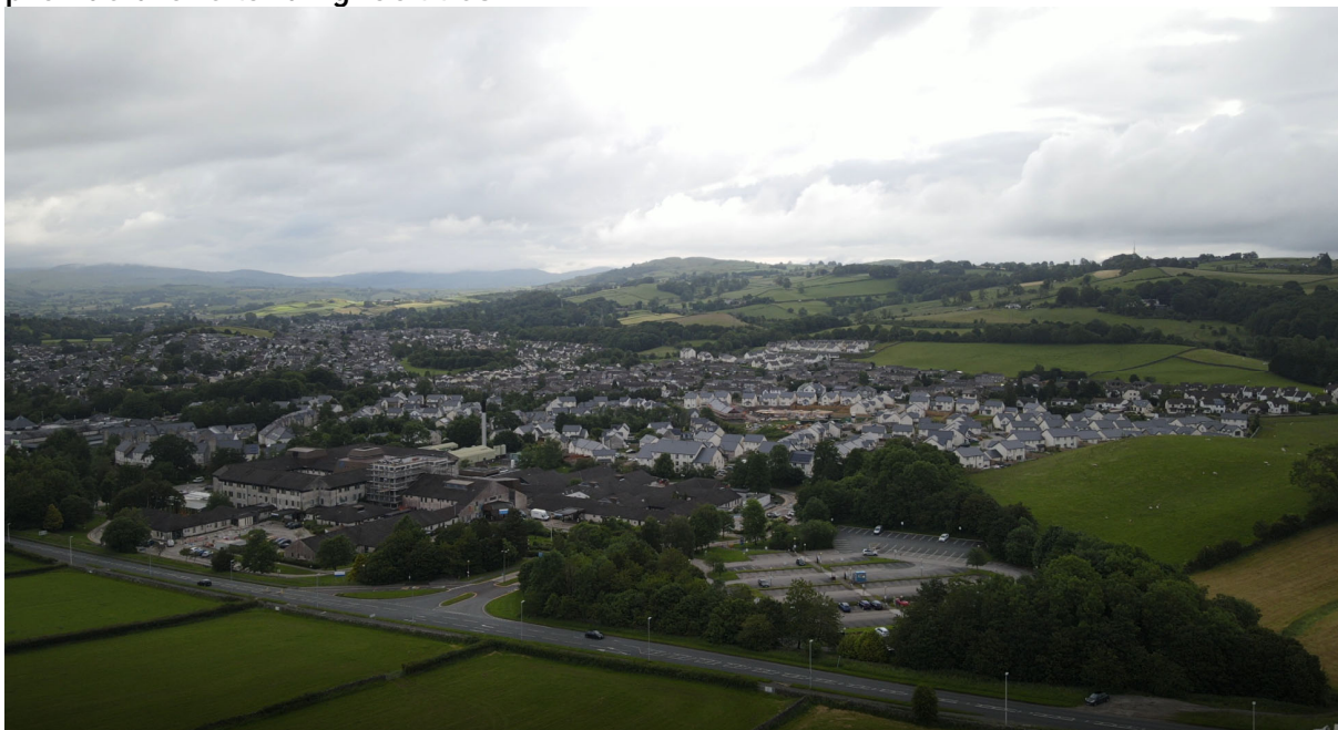
Figure 6.14 – The approach into Westmorland General Hospital
