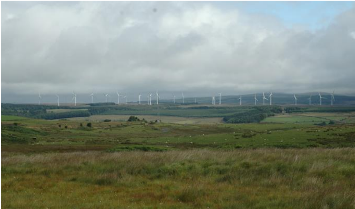
Figure 2: Mark Hill windfarm
