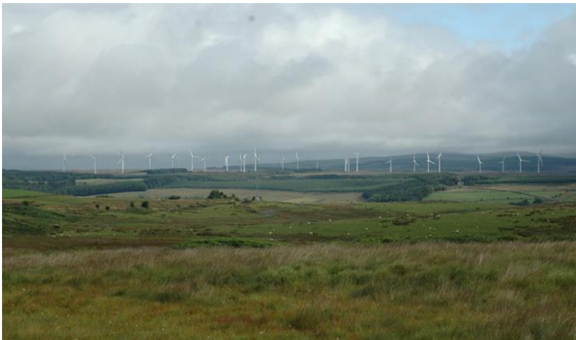
Figure 1: Mark Hill windfarm
