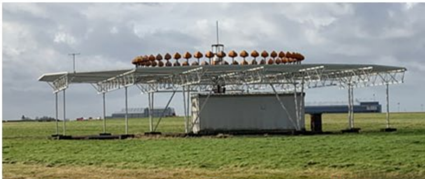
The Manchester Doppler VHF Omni-directional Range (MCT DVOR). A ground-based radio navigation beacon used by pilots to assist in aircraft navigation.
